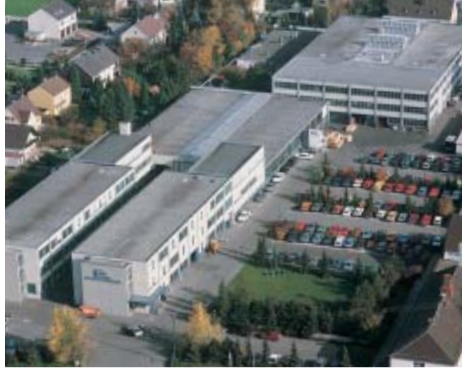
Head office E+L Augsburg Germany
